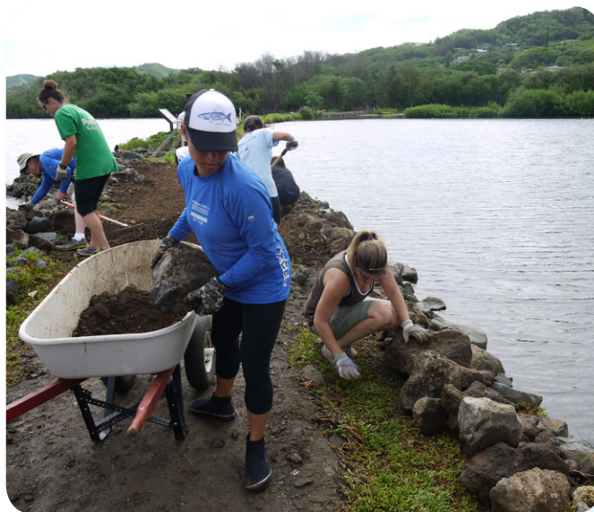
Restoring the rock wall at Waikalua Loko Fishpond
