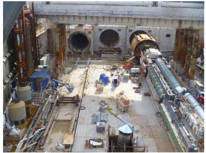
Figure 12. Tunnel Boring Machine
