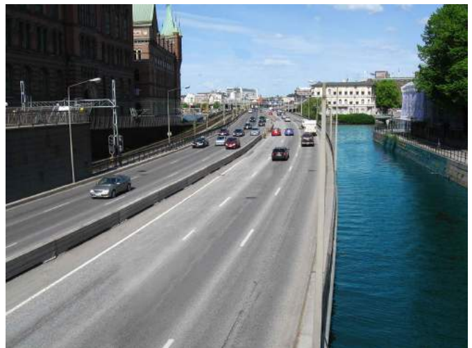
Figure 48. Bridge Next to an Urban Waterway
