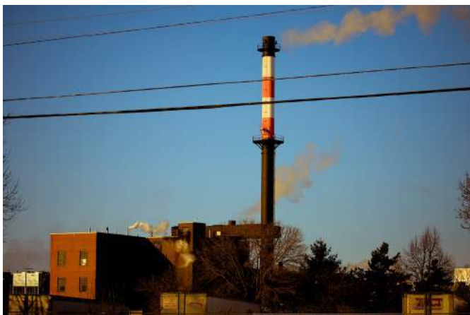
Figure 4. Smoke Trapped Between Wires
